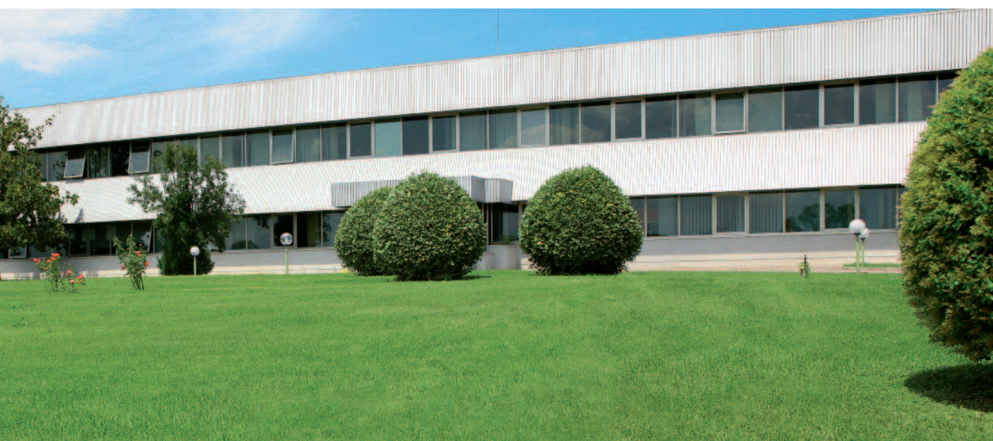
Castelfidardo plant - Italy
